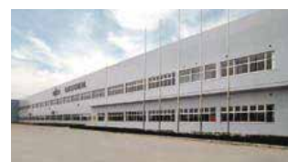
Fujitsu General Central Air-conditioner (Wuxi) Co., Ltd.
