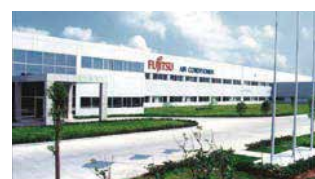
Fujitsu General (Shanghai) Co., Ltd.
