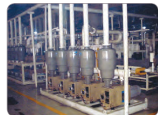
Helium leak test
